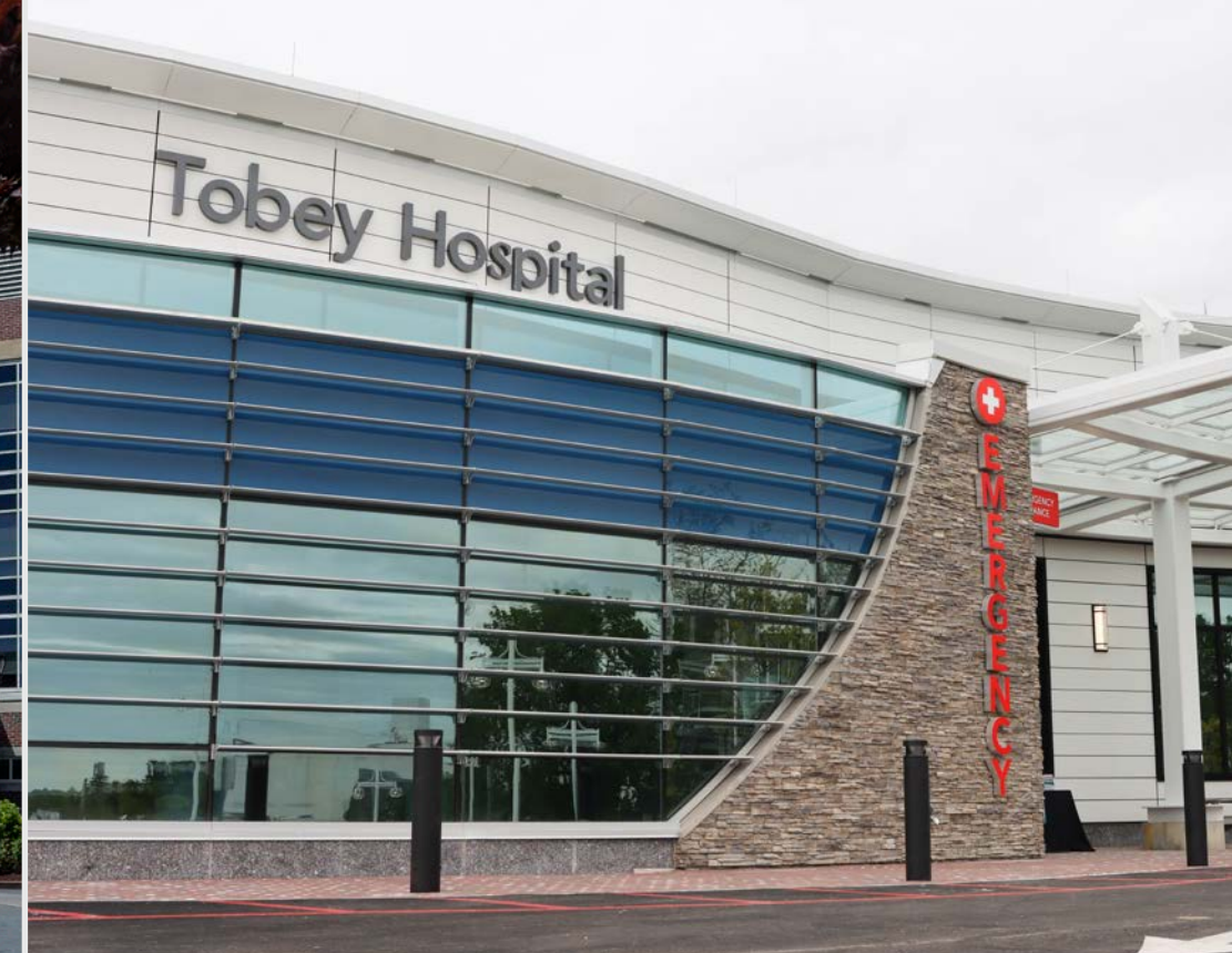
Tobey Hospital – Wareham, MA
