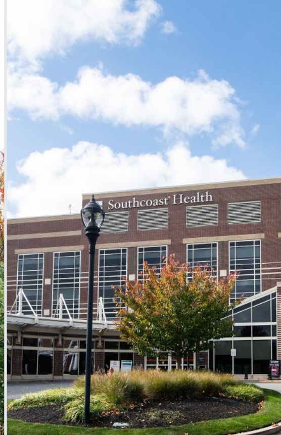
St. Luke's Hospital – New Bedford, MA
