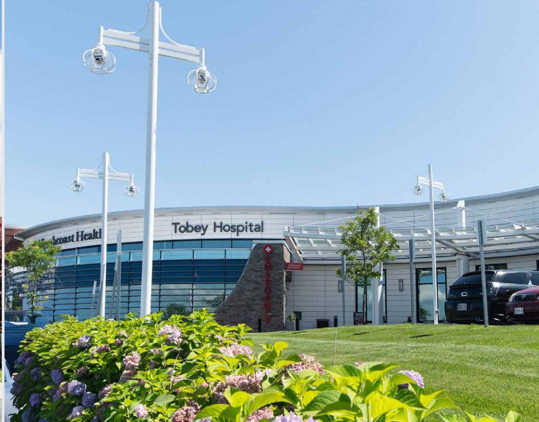
Tobey Hospital – Wareham, MA
