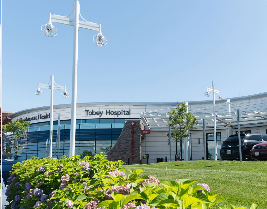
Tobey Hospital – Wareham, MA
