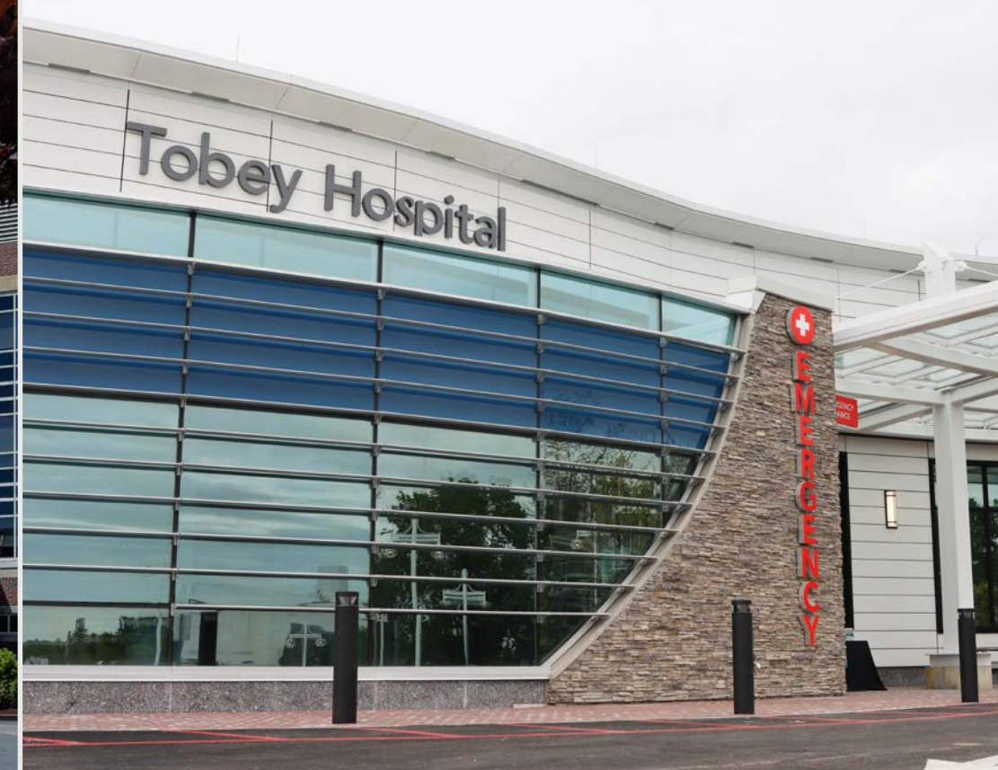
Tobey Hospital – Wareham, MA
